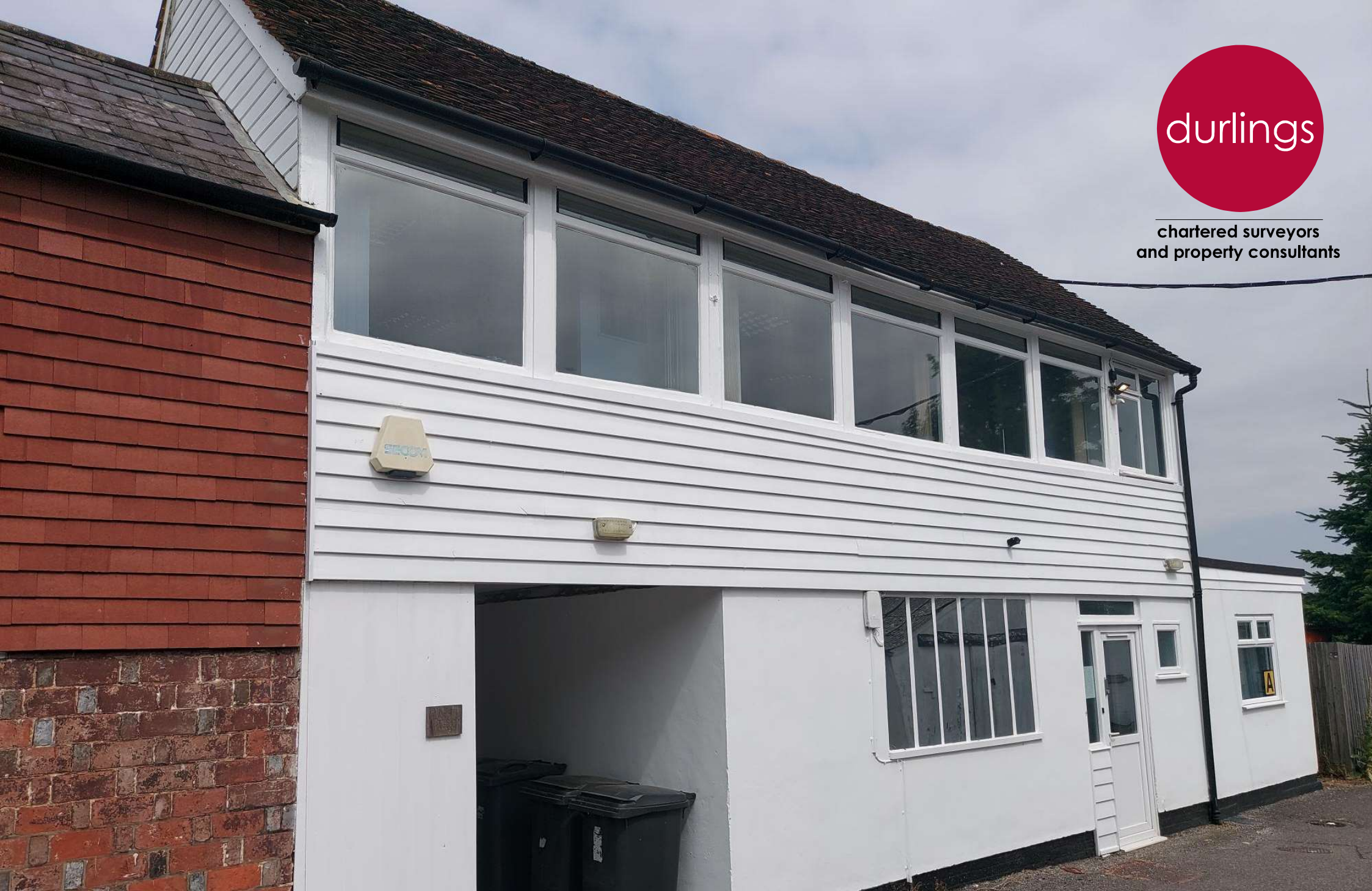
Unit A Durgates Industrial Estate • Durgates • Wadhurst • East Sussex TN5 6DF Refurbished Office Building To Let - 589 sq ft (54.67 sq m) – net internal
